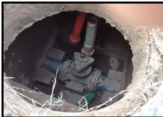
Fire hydrants as pipe insertion point
