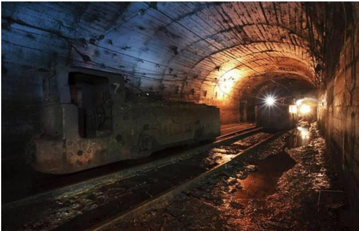
Figure 2: A typical coal mine tunnel
