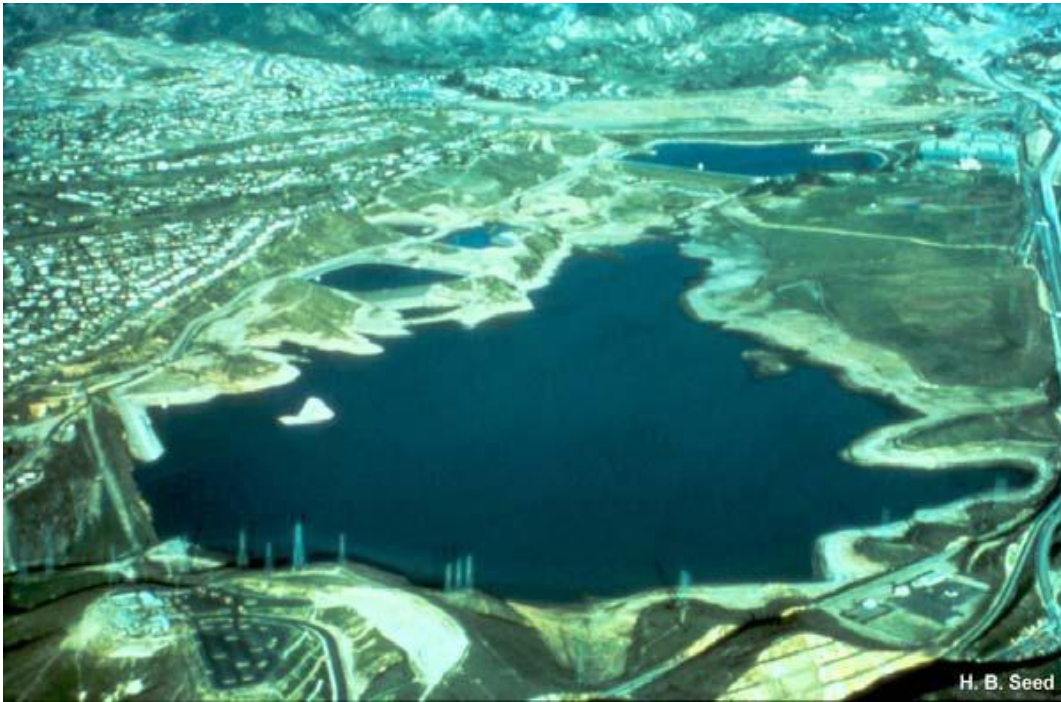
General View of the Site
