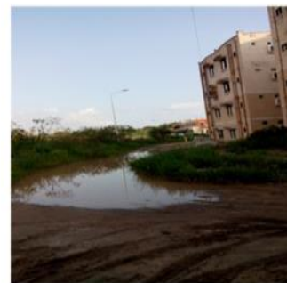
6. No Proper Rainwater Disposal
