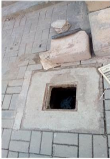
8. Open Main Holes
