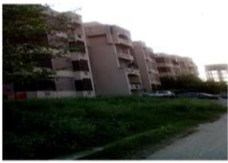
6. No Parking Place
