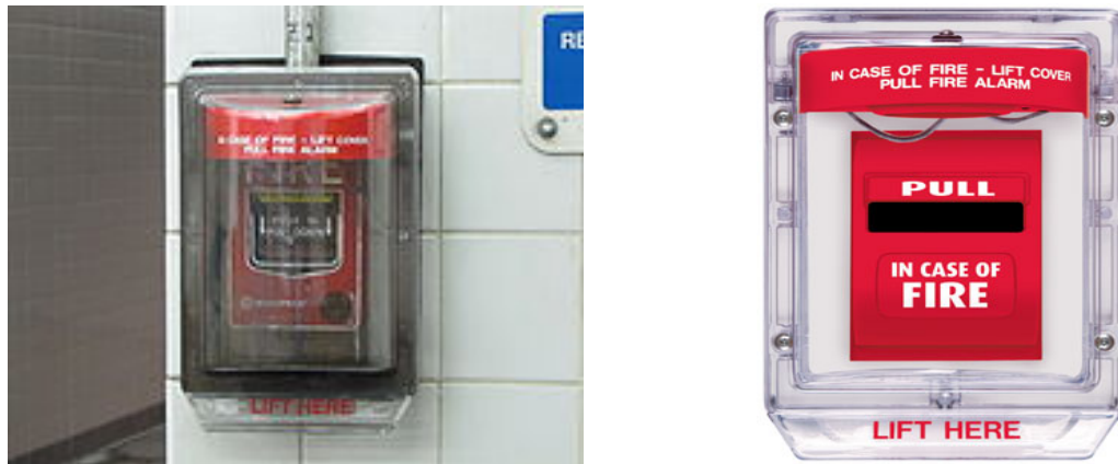
Figure 2 – 4 Pull Station Fire Alarm
