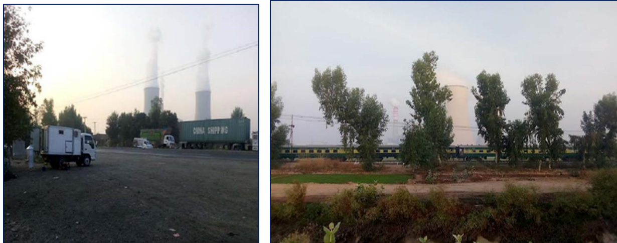
Surroundings of Sahiwal Coal Power Project.
