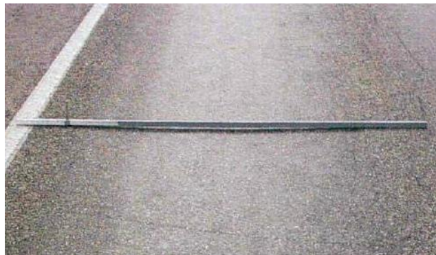
Figure 2. 13 Permanent Deformation in Pavement
