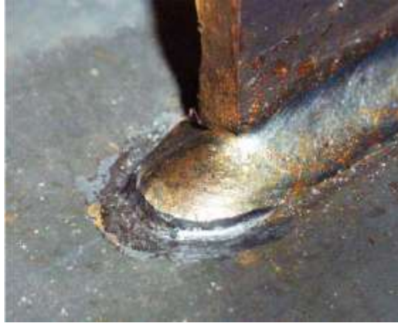
Figure 3: Air hammer peened weld toe [2]
