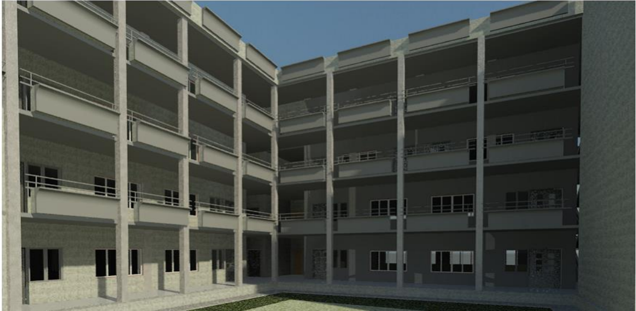
Figure 9: Back side of the building
