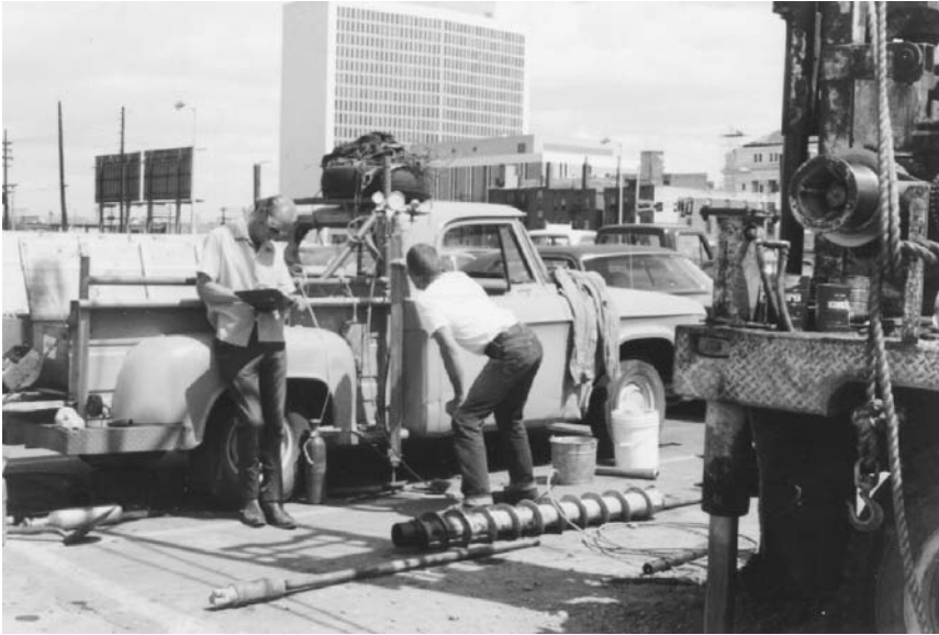
FIGURE 3.1 Drilling for pressuremeter test.
