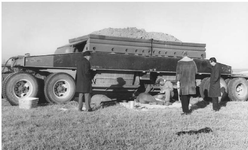
FIGURE 3.7 Plate bearing test for the construction of runway.
