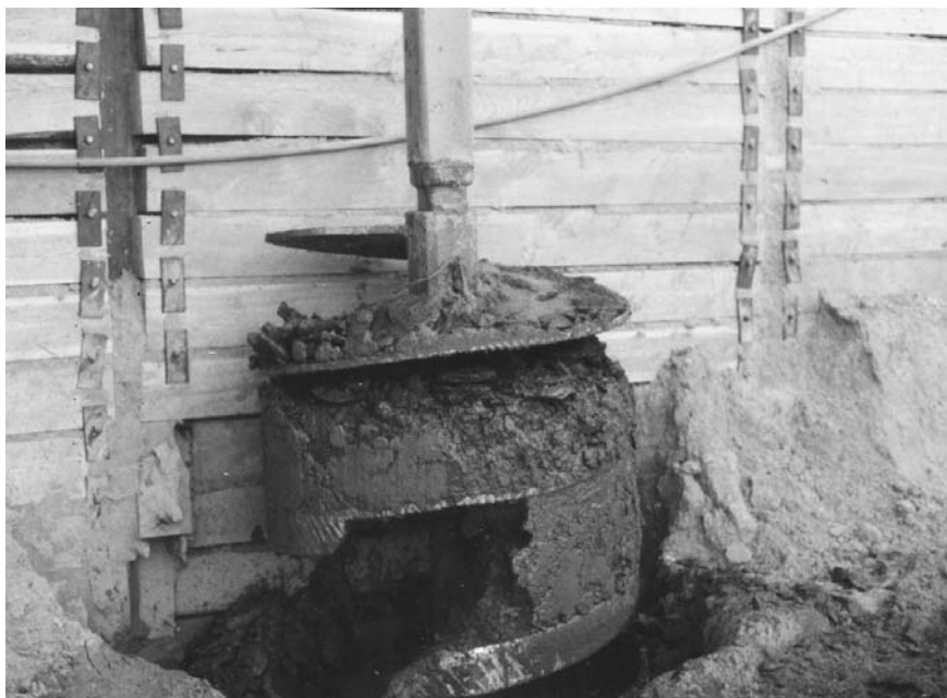
FIGURE 10.3 Large-diameter pier drilling for a high-rise building.
