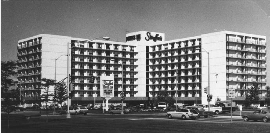
FIGURE 9.3 Stouffer's hotel, built with footings on compacted fill.
