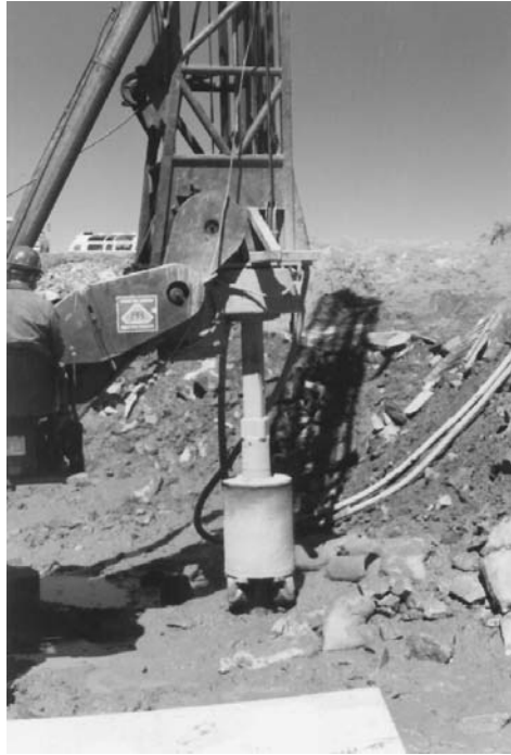
FIGURE 2.1 Caisson rig with a rock bit.
