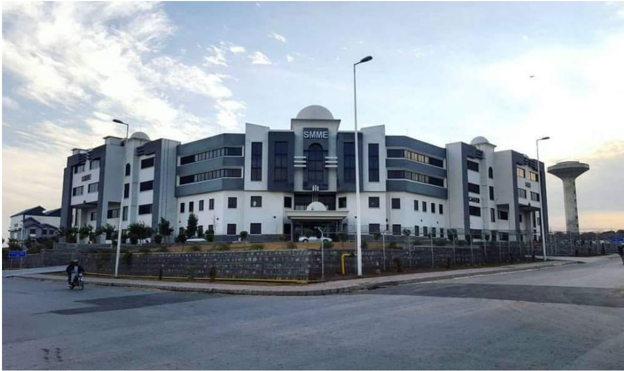
Figure 4: Front view of SMME building
