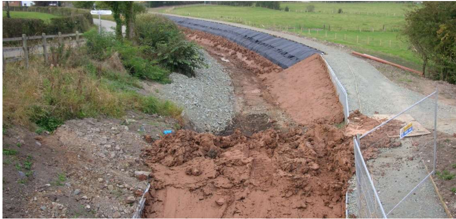
Figure 2.6 Puddle Clay Lining being applied to Montgomery Canal, England
