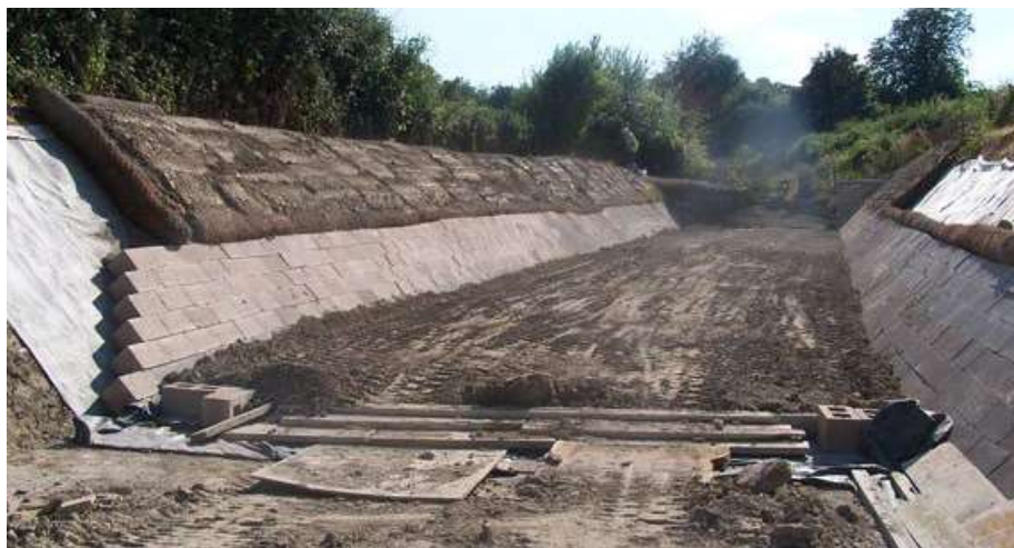
Figure 2.7: Brick Lining being applied to a canal
