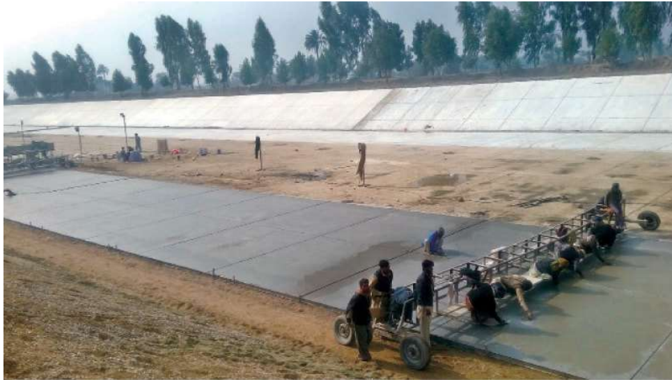
Figure 2.8: PCC lining being applied to Muzzafargarh Canal, Pakistan
