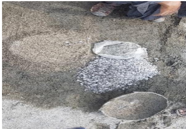
Figure 18: Mixing in cement and prep of mortar
