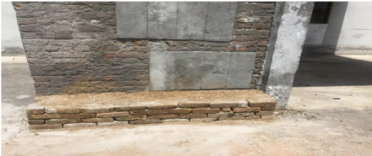
Figure 16: Construction of Platform
