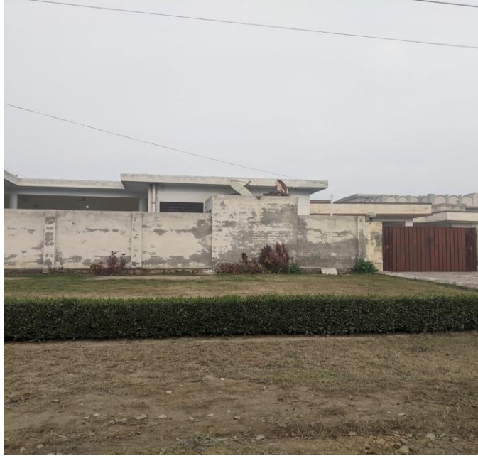
Figure 12: Residential wall opposite Farhad Sports Complex
