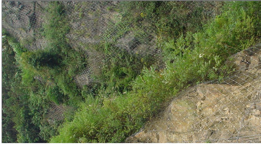
Figure 3.8: Flexible Prevention Mesh
