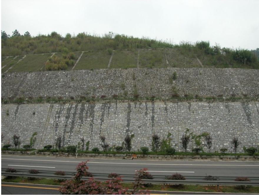
Figure 3.4: Mortar Rubble Slope Protection
