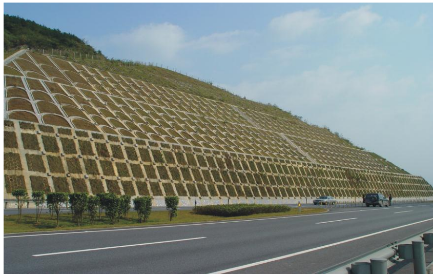
Figure 3.7: Reinforcement Works of Prestressed Anchor and Frame Girder
