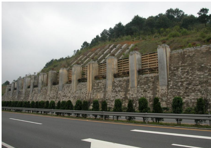
Figure 3.1: Anchor pile
