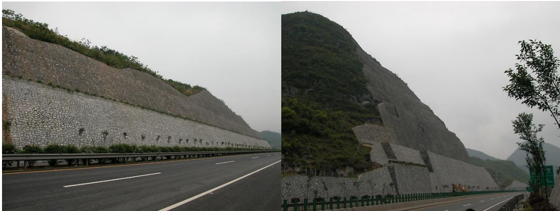
Figure 3.5: Face Protective Wall
