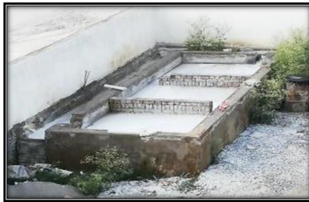
(Figure 16. Existing Sedimentation Tanks)
