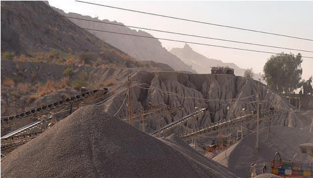
Figure 3.2: Margallah Hills Crush Plant
