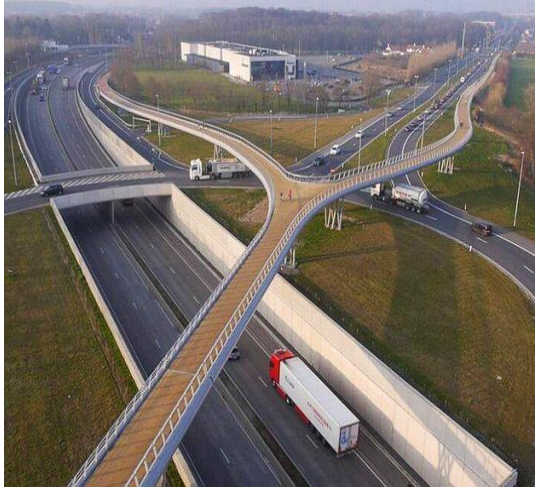
Figure 5. 11: Bridge above road
