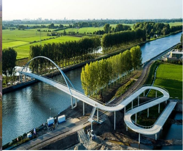
Figure 5. 10: Bridge above canal
