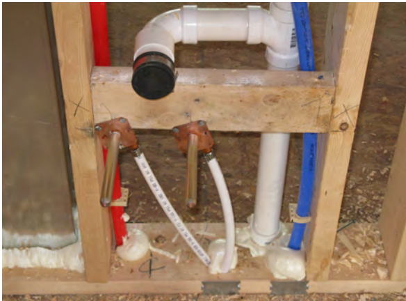
Plumbing penetrations between floors.
