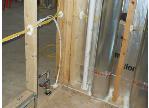
Plumbing, electrical and HVAC penetrations between floors.
