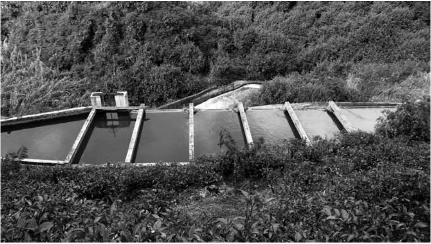
Figure 8.5 An abandoned 2.5 MW grid-connected mini-hydro system at the Carolina Tea Estate, Sri Lanka
