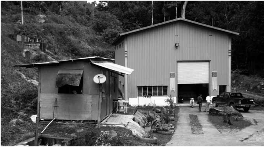
Figure 11.1 The 2 MW Kerling minihydro plant, Malaysia
