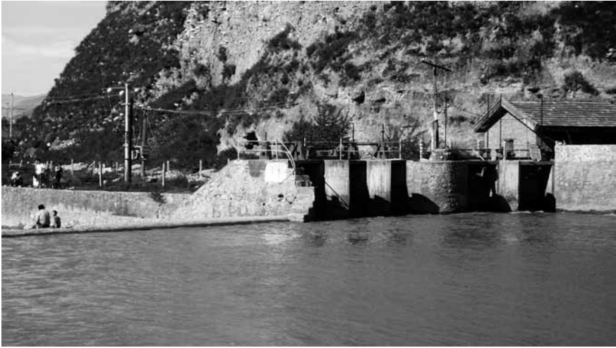
Figure 4.6 A 16.5 kW Grid-connected small hydro facility near Rebgong, China
