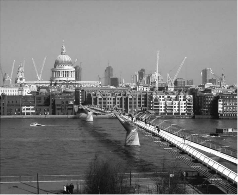
Fig. 13.10. The Millennium Bridge in London (courtesy of Arup).
