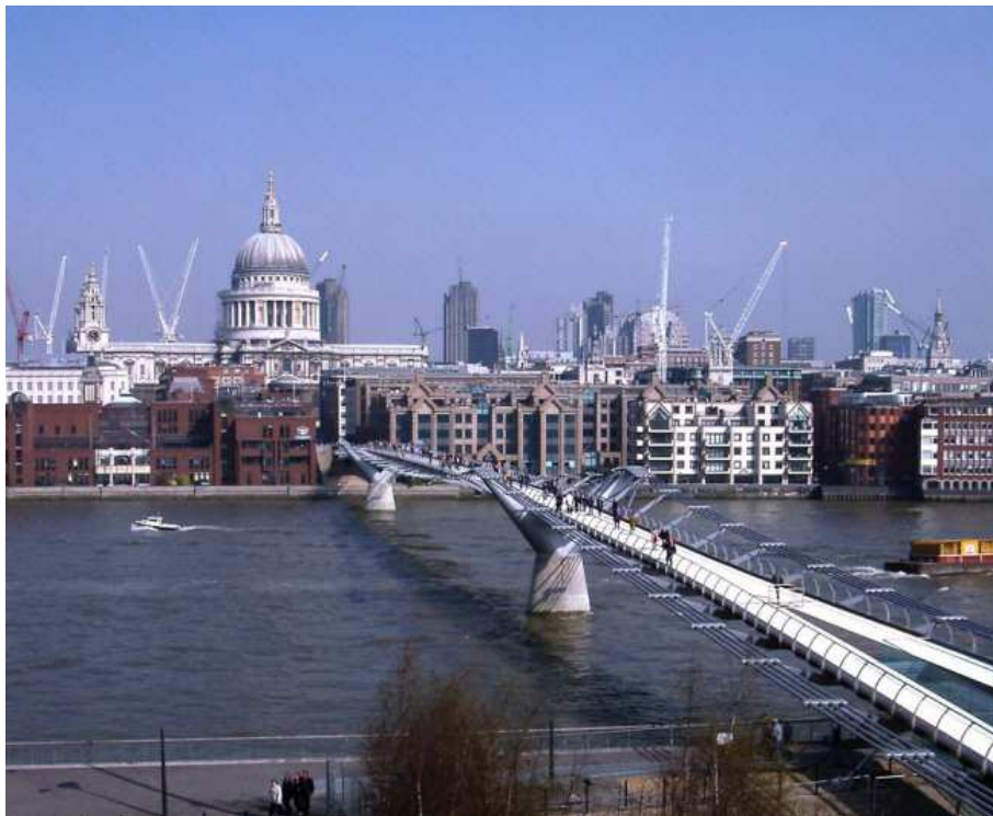
Fig. 13.4. The Millennium Bridge in London (courtesy of Arup).
