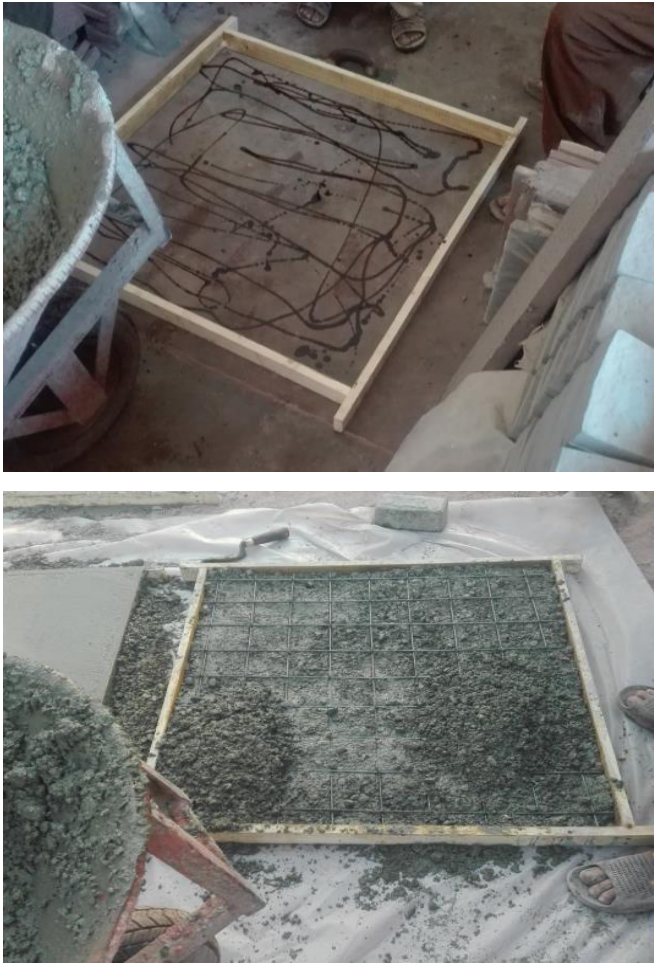
Figure 20: Pouring of concrete
