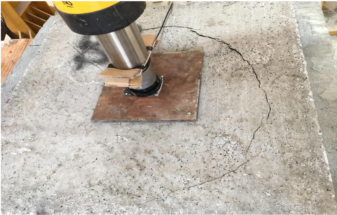
Figure 28: Cracking Pattern of Reinforced slab
