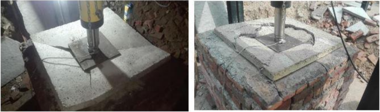
Figure 7: Testing of Poly-urea Coated Slabs
