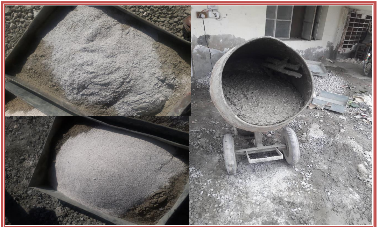
Figure 7 Mixing of Concrete Ingredients
