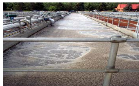
Figure 2.4: Foaming in activated sludge process
