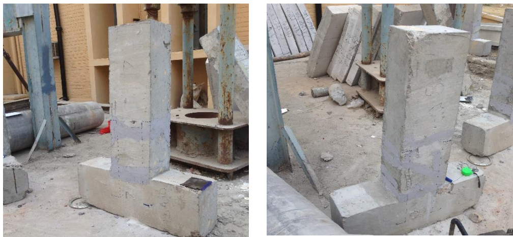
Figure 3.2 Joints repair work using non-shrink grout Chemdur-31
