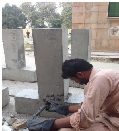
Figure 3.3 Filling of joint cracks using resins
