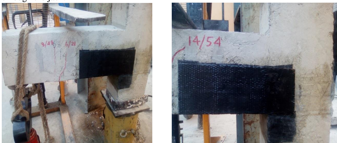
Figure 3.6 Joints repaired using CFRP
