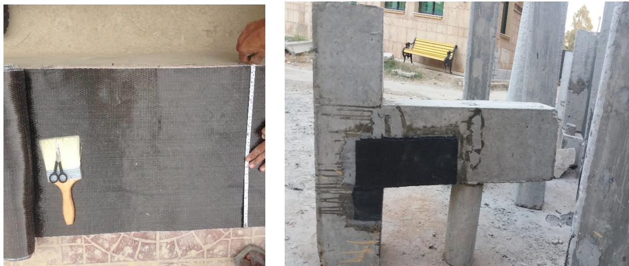
Figure 3.4 CFRP being applied to damaged specimen
