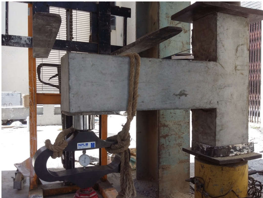
Figure 22: Collars Installed at Column Ends
