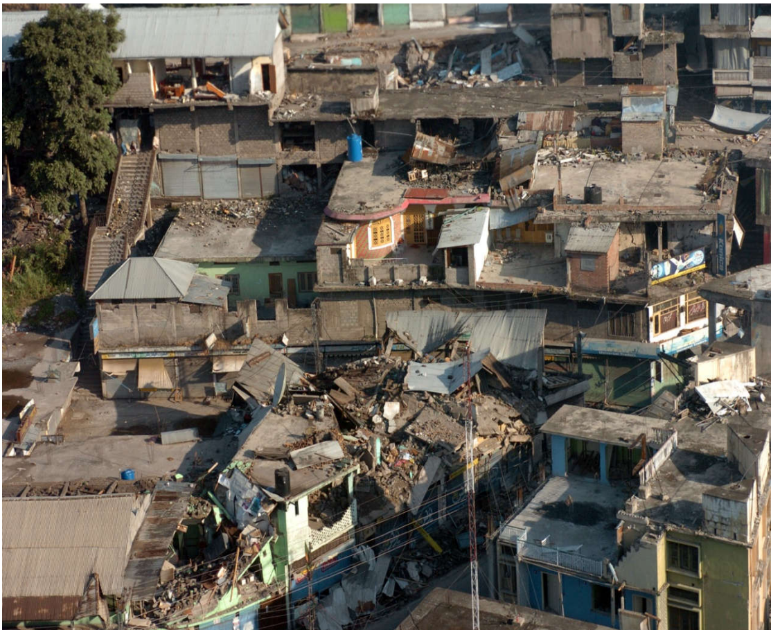
Figure 2: Earthquake Destruction in Muzaffarabad - 2005
