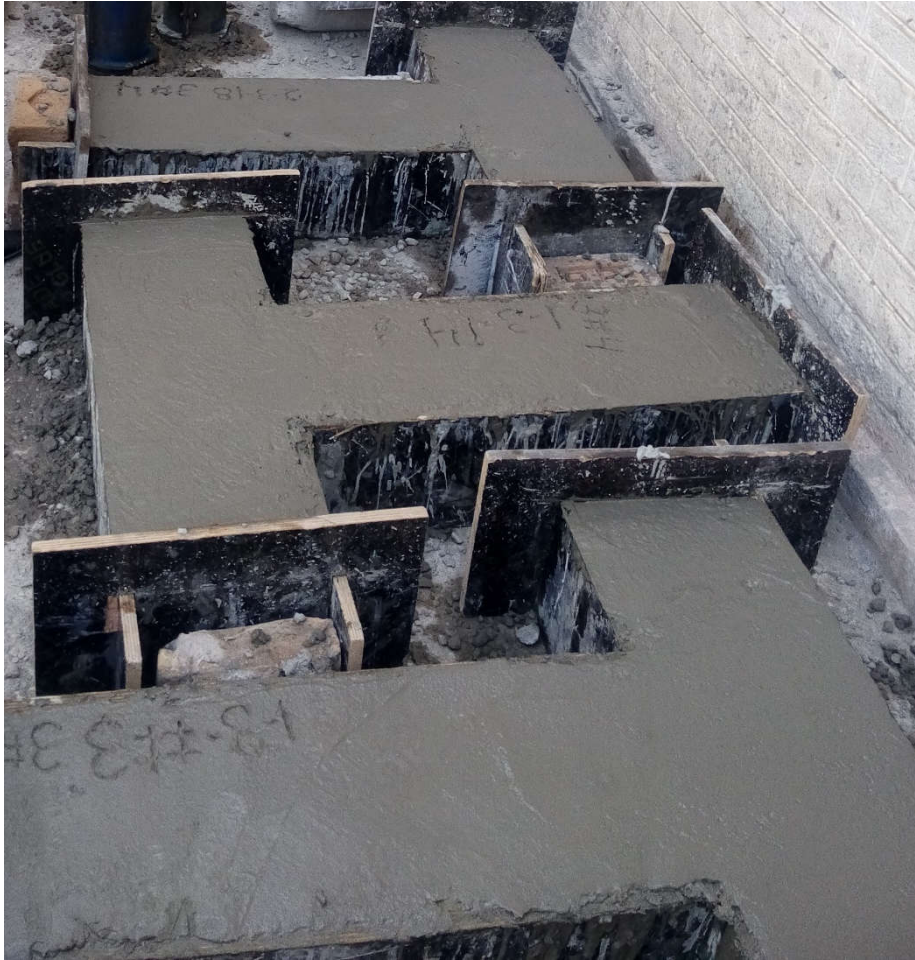
Figure 15: Casting of Specimen
