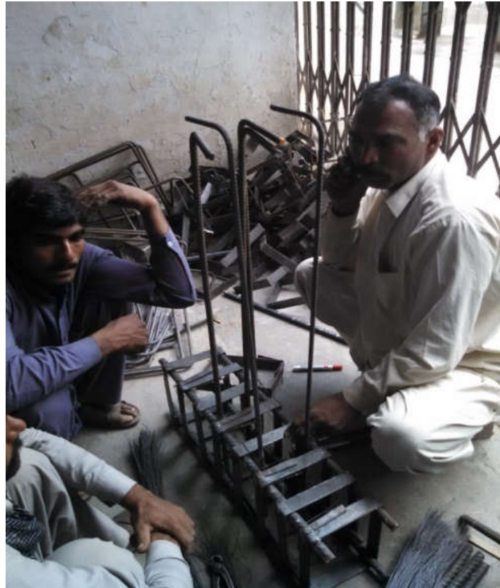
(a) Construction of steel cages
