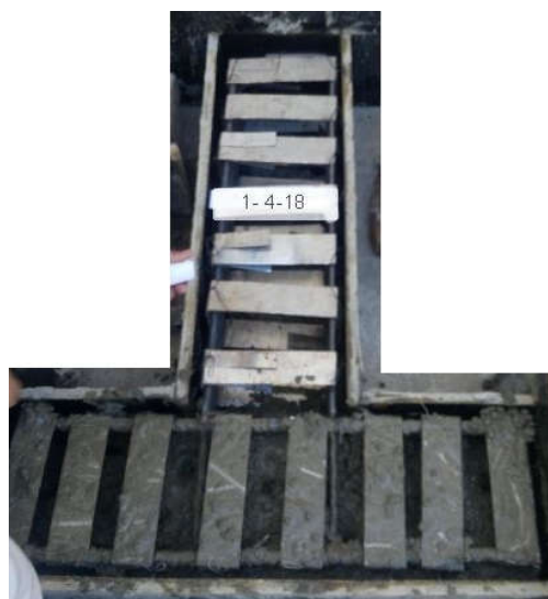
Figure 14: Joints before Casting
