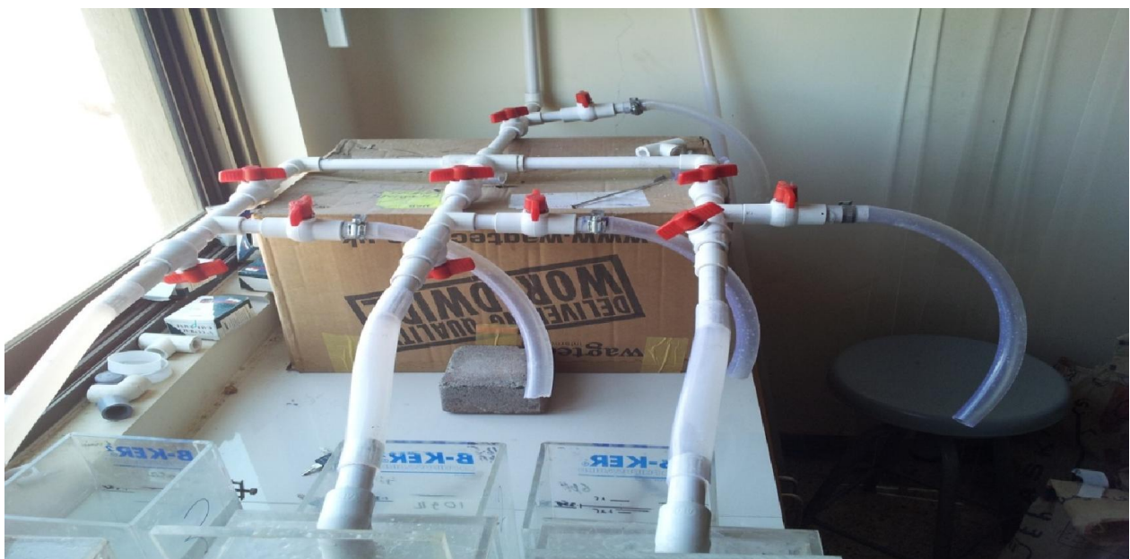
Figure 3-4: Valve and pipe assembly used to control the flow rate
