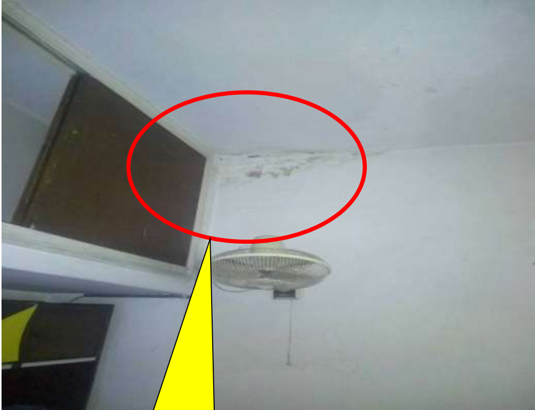
Rotting & Wrapping of Timber
