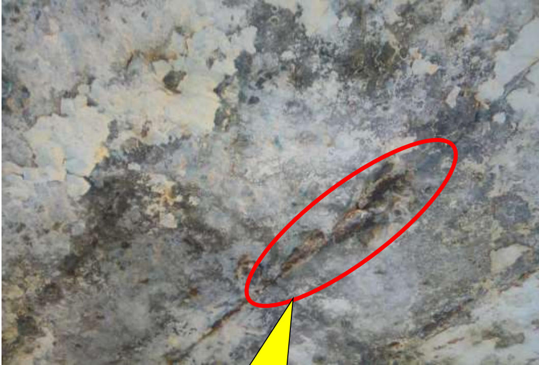
Corrosion of Reinforcement
