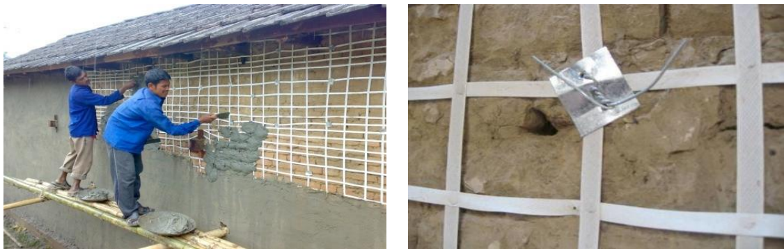
Fig 2.16 Application of PP-meshing
