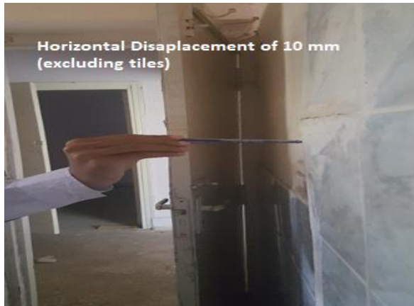
(c) Bathroom attached to Bedroom 2
