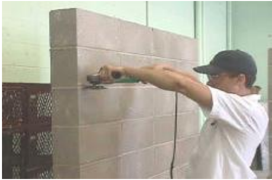
(a) Grinding of mortar joints
