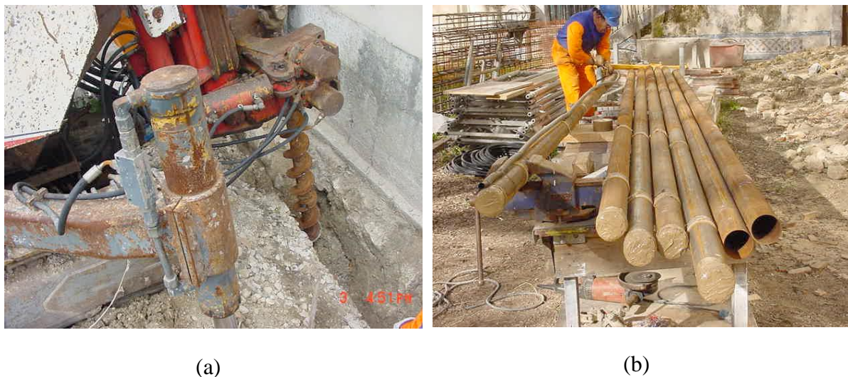
Fig 2.12 (a) Micro pile drilling machine (b) Micro pile casing
