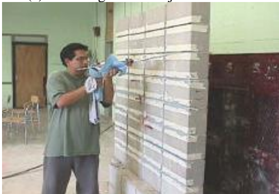
(c) Injection of epoxy paste
