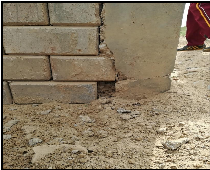
Figure 4. 14 Bulging of wall after blast test
