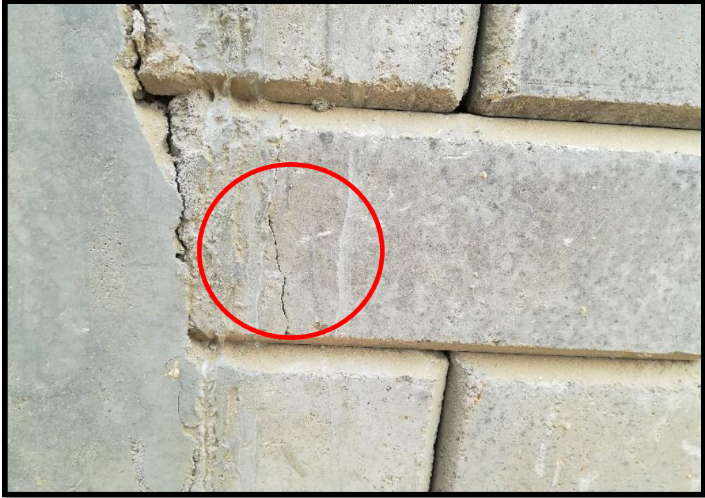
Figure 4. 8 Hair line cracks in the blocks.
