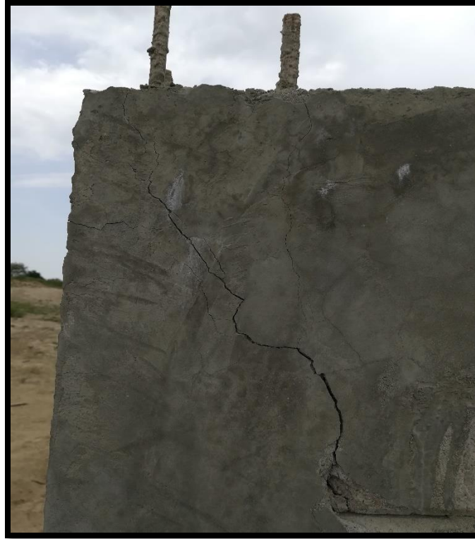
Figure 4. 16Cracks at the joint Horizontal and vertical confinement element.
