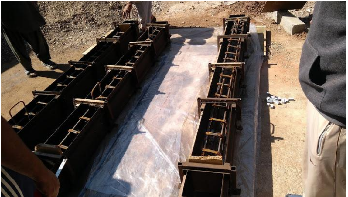
Figure 4-4: Placement of reinforcement into the molds
