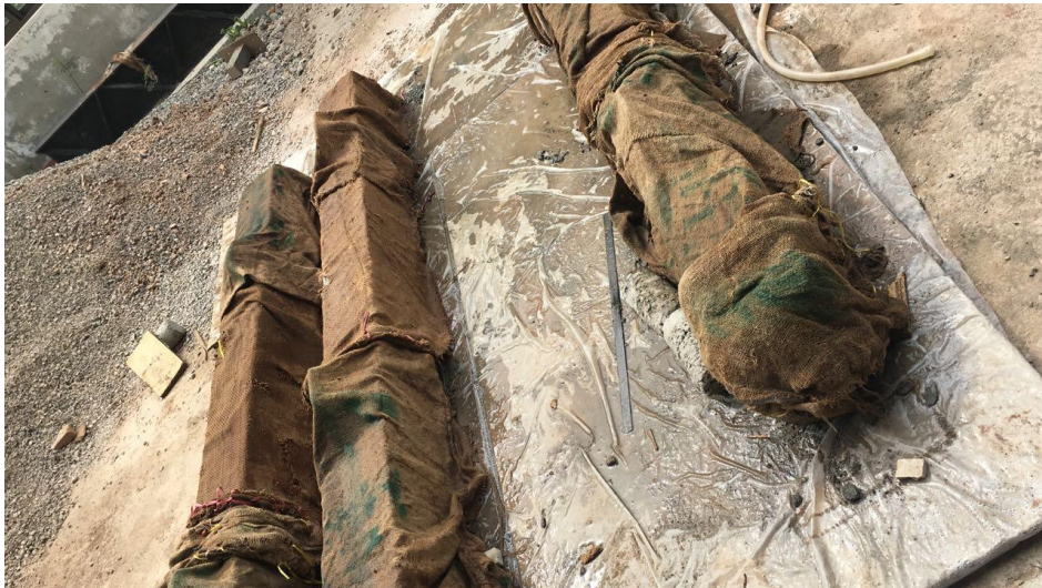
Figure 4-5: Curing of beams
