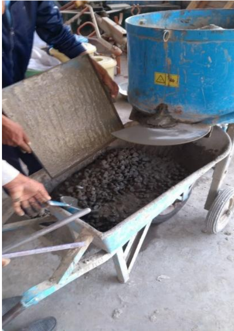
Figure 4-3: Mixing in the batching unit
