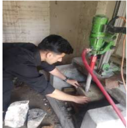
Figure 4-22 Rock core extraction
