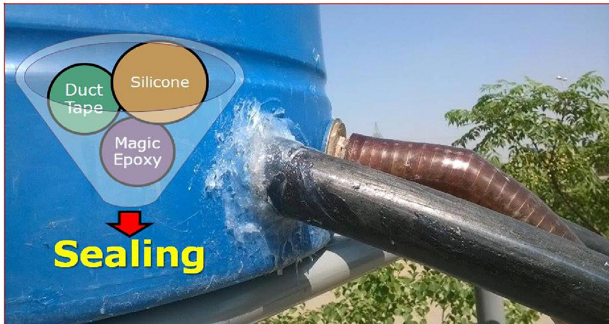
Figure-21 Sealing using silicone sealant.
