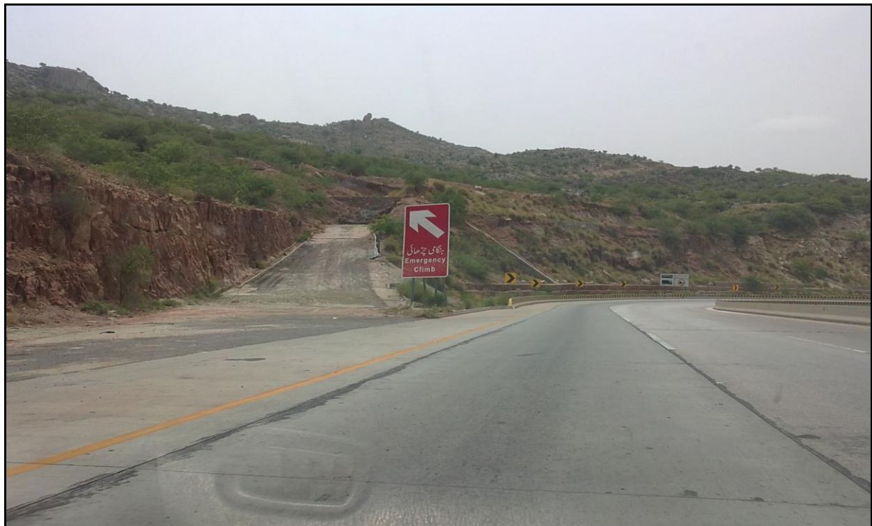
Figure 5.13: Motorway Emergency Climbing Ramp
