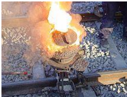
Fig 1.7 Thermite reaction proceeding for a railway welding. Shortly after this, the liquid iron flows into the mould around the rail gap
