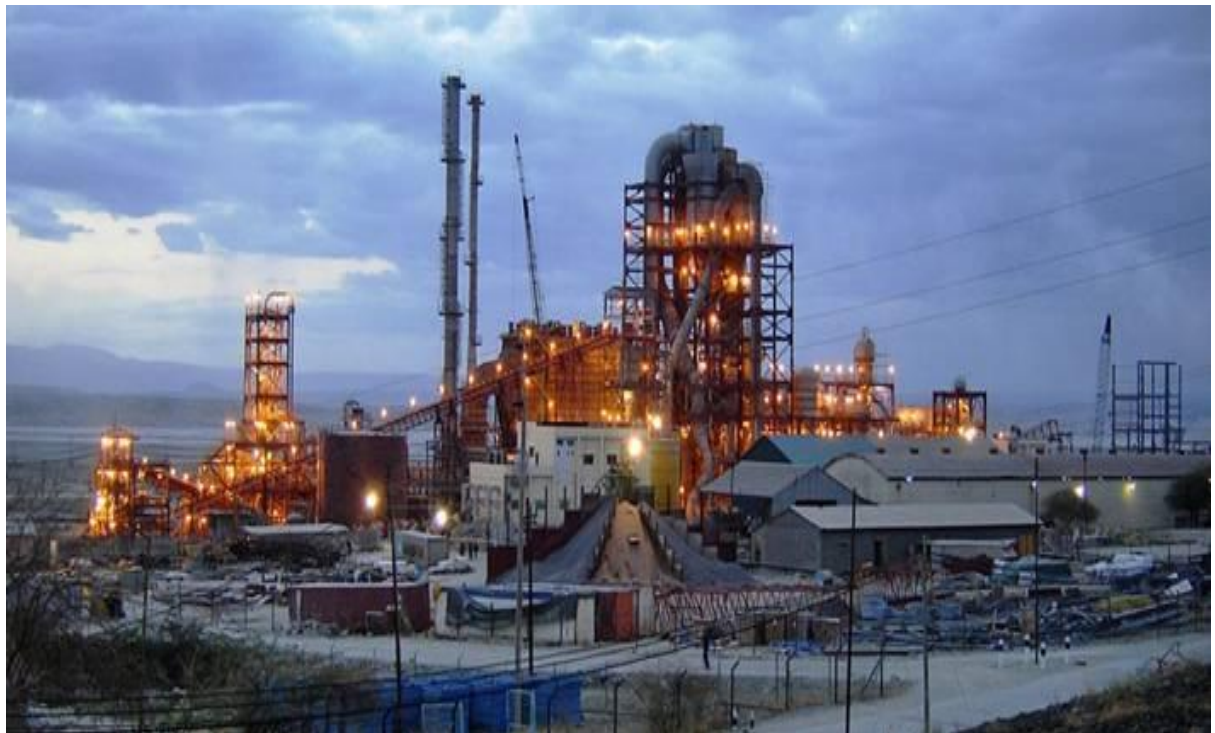
Figure 1 ICI Soda Ash Plant
