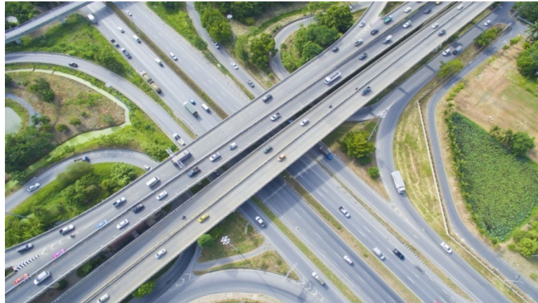
Figure 2.3 Images Showing an Overpass
