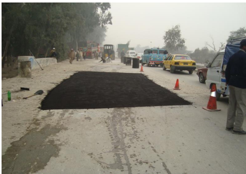
Fig.1.2. Expansion project of Ring Road Peshawar
