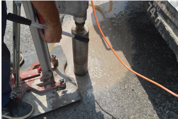
Figure 3.6: Core Cutting Process
