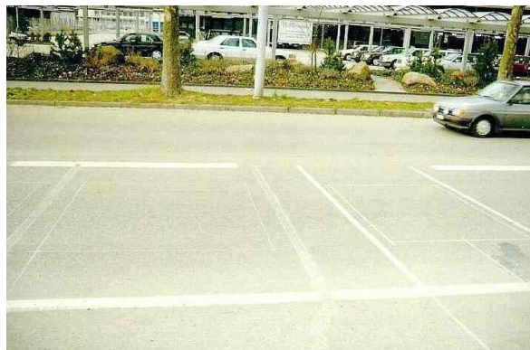
Installed Piezo Quartz WIM
