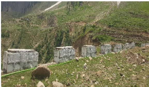
Figure 4.34: Installed Barriers along the edges (Also Broken from corners i.e. Burhwai)
