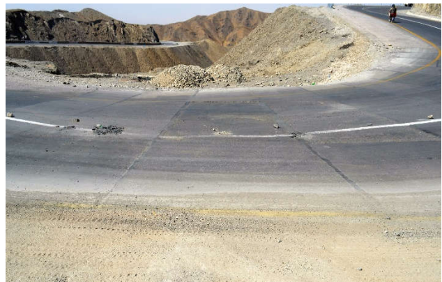
Figure 4.26: Causeway constructed (Enroute Naran)
