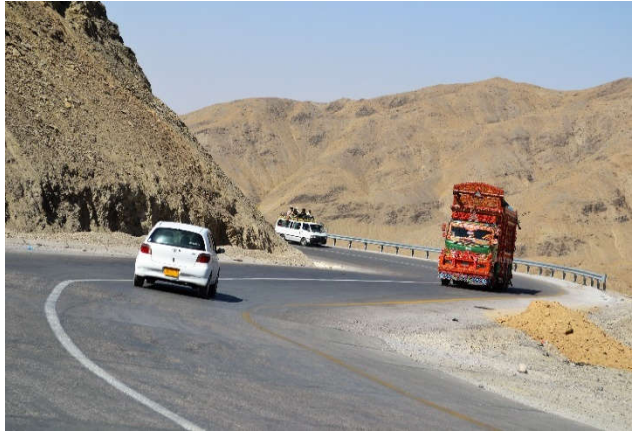
Figure 4.25: illustrates problem with vehicle negotiating the curve (Batakundi) Note: car has encroached into opposite traffic lane
