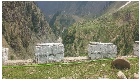
Figure 4.34: Installed Barriers along the edges (Also Broken from corners i.e. Burhwai)
