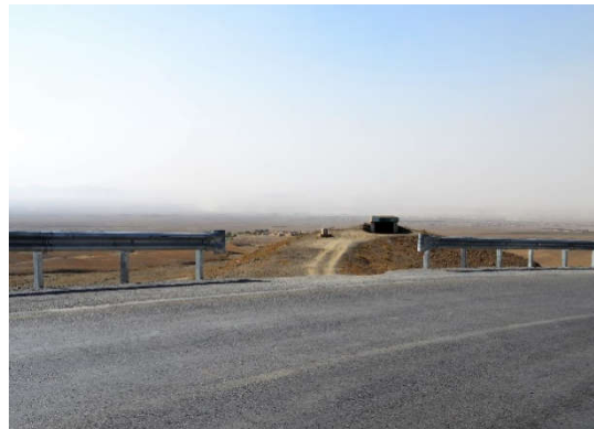
Figure 4.30: illustrates the discontinued guide rail (Naran)
