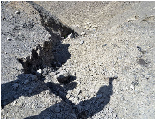
Figure 4.27: illustrates the erosion problem (non-project)
