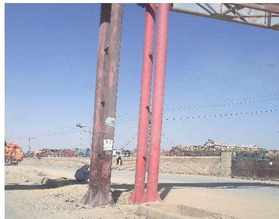
Figure 4.16: Existing gantry sign post on N-15.
