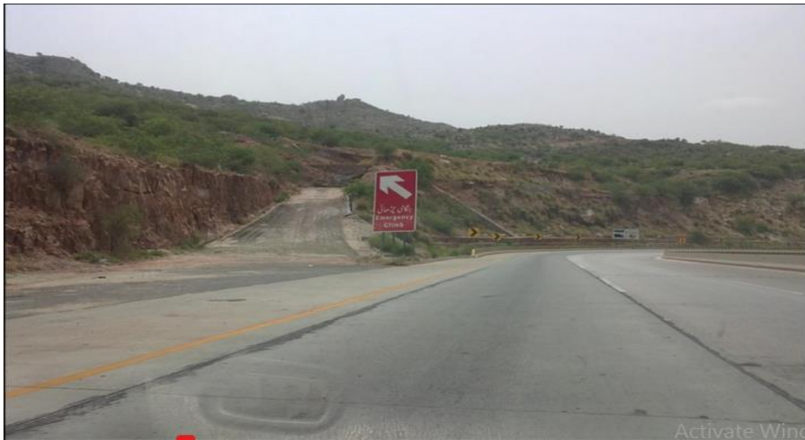
Figure 5. 4: Climbing ramp provided to prevent brake failure.
