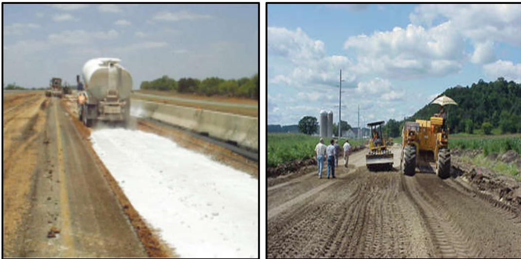
Figure 1-1 (a,b) Practical Application (a) Lime and (b) fly ash in Subgrade Stabilization
