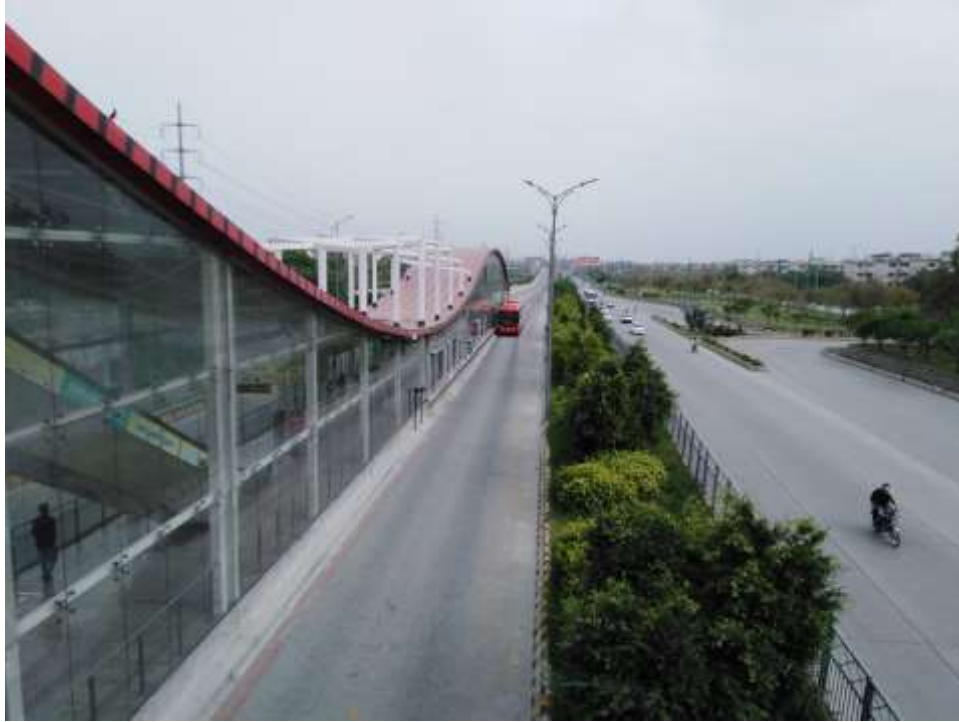
Figure 2.3: Fencing along the corridor of PMBS
