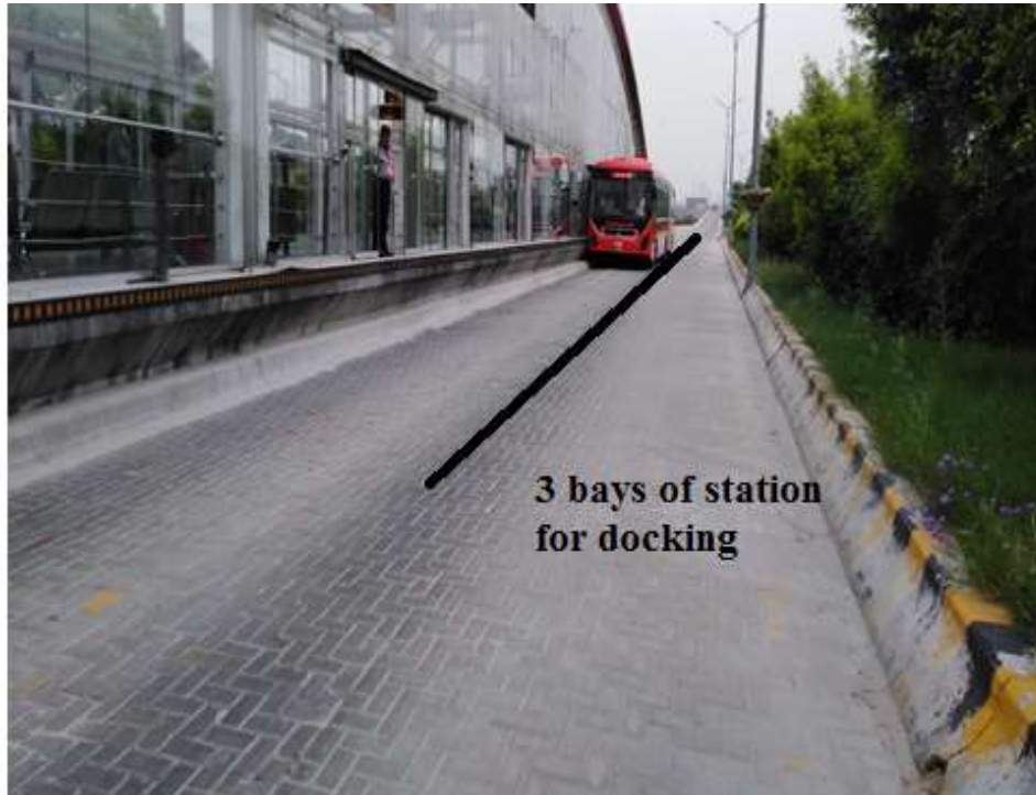
Figure 2.6: 3 Docking Bays of PMBS Stations
