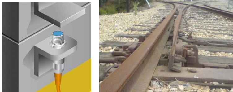
Figure 3.2: Detection of point setting by inductive sensor [31][36]
