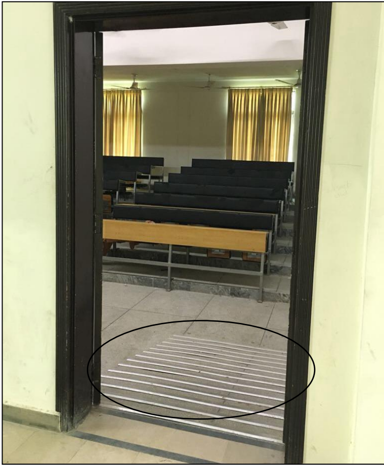
Picture 4.13: Ramp for entering the classroom in the Department of Natural Sciences at Quaid-e-Azam University
