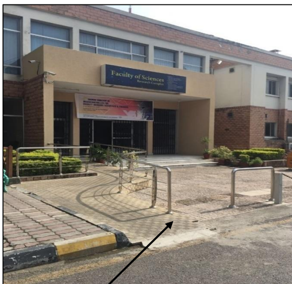
Picture 4.5: Ramp in Faculty of Science Department, QAU
