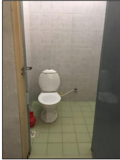
Picture 4.15: Accessible Washroom in Faculty of Engineering & Computer Sciences, NUML University
