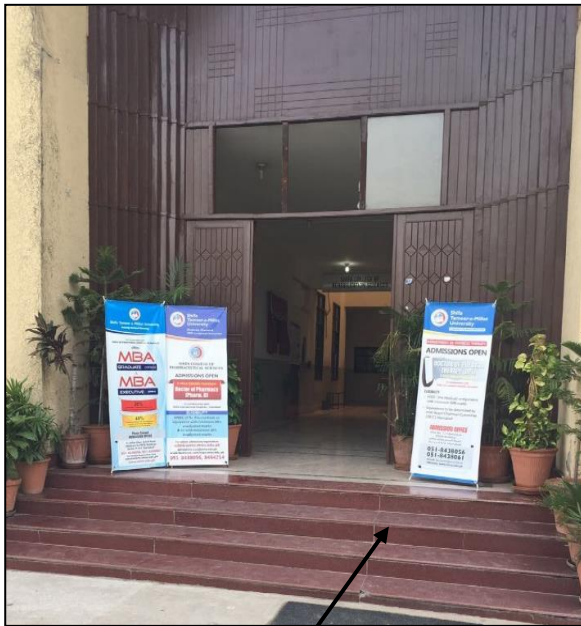
Picture 4.3: No Ramp in STMU
