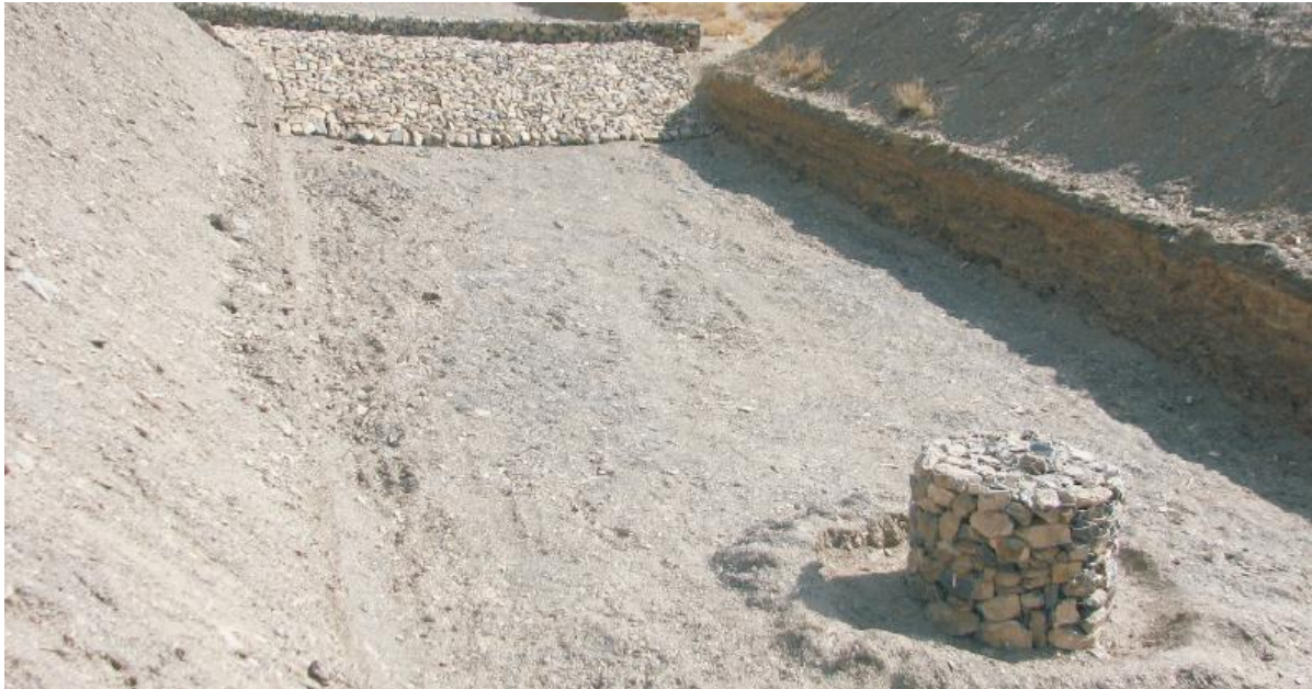
Figure 2- 6: An Inverted well on the upstream of a leaky dam (Source: Sustainable groundwater Management in Baluchistan)
