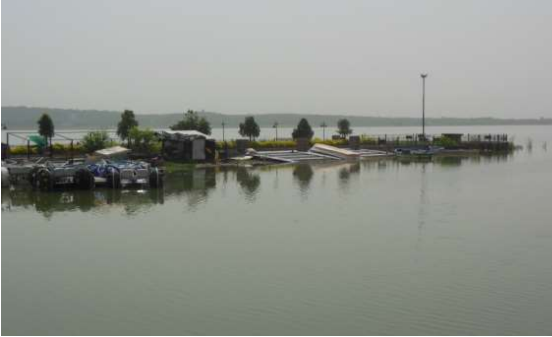
(15) LOCATION OF SITE RAWAL DAM
