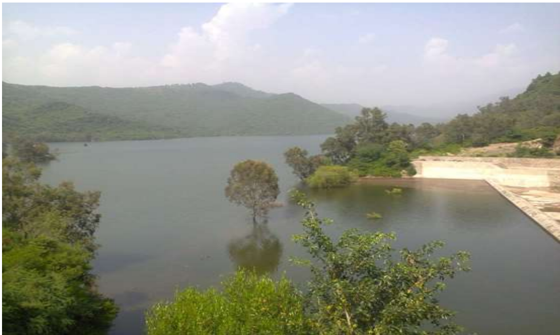
(14) LOCATION OF SITE Simly DAM
