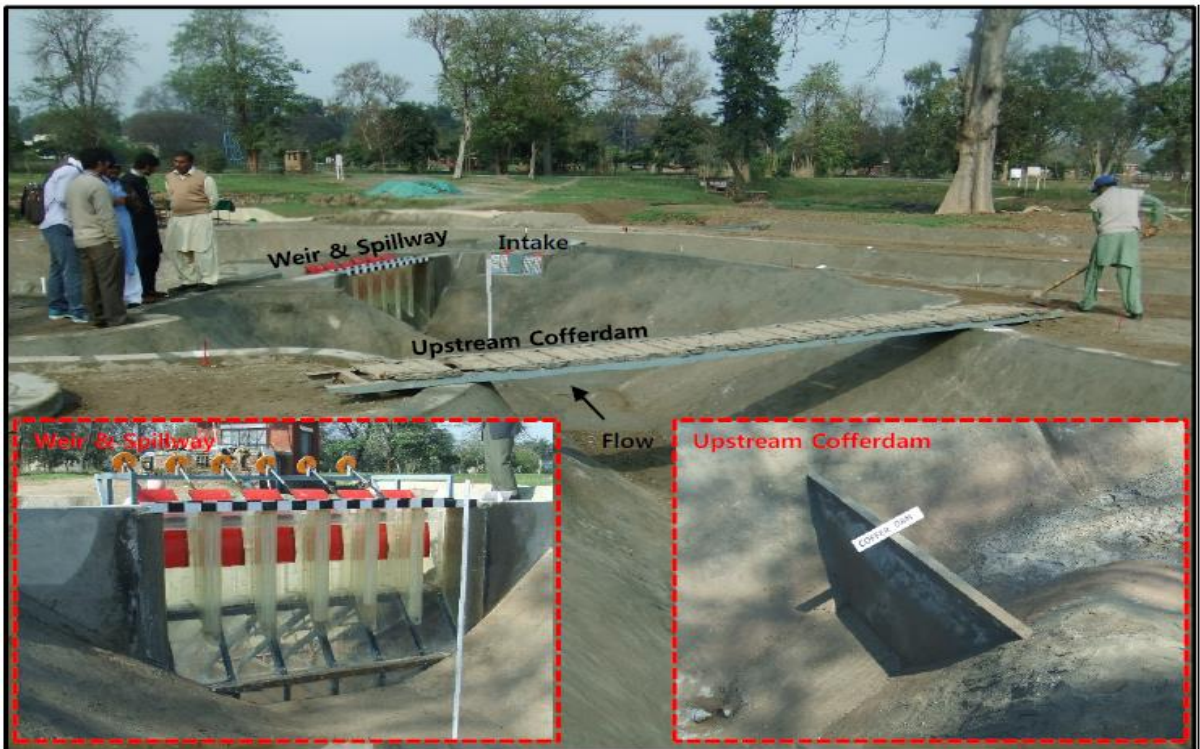
Figure 4.2: Weir upstream view
