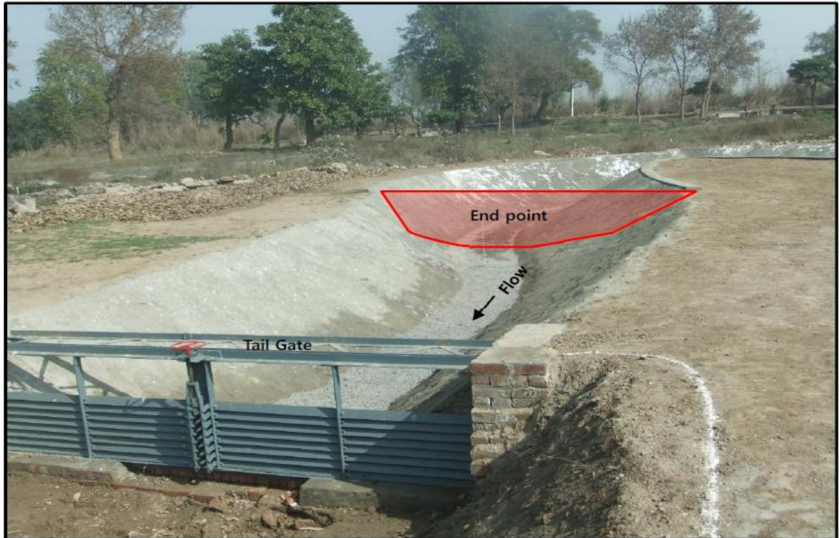
Figure 4.4: Tail gate arrangement
