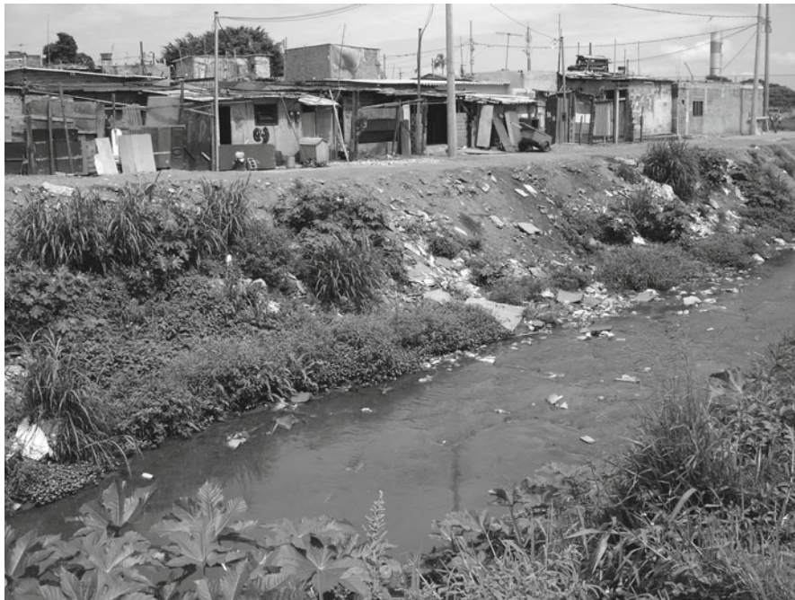
Fig. 8.6 Slum area located at the edge of watercourse: example of association between exposure to environmental risk and precarious socioeconomic conditions in São Paulo City (Photo by Luciana Travassos)
